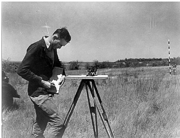
Figure 8: Chain and compass for surveying (above) and plane tables (below) – very common through until late 1960's
