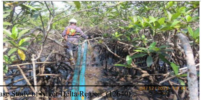
Discovered Siphon Hoses Destroyed During Pipelines ROW Surveillance
