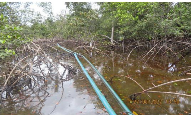
Illegal Siphon Hoses Discovered During Pipelines ROW Surveillance
