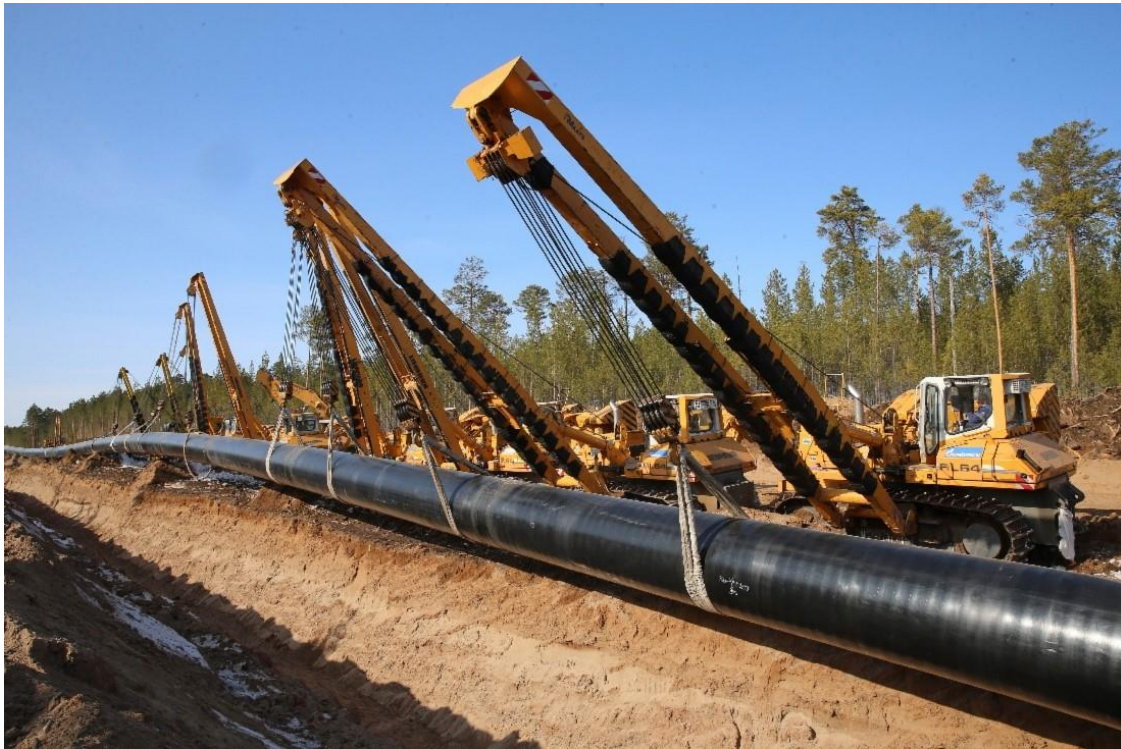
Figure 3: Part of the 210 km onshore pipeline across Denmark being established
