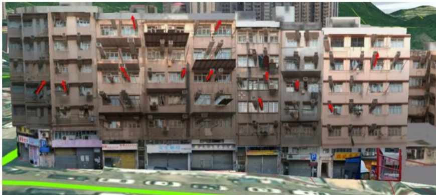
Figure 7: Texture of Building Façade Skewed in Different Directions
