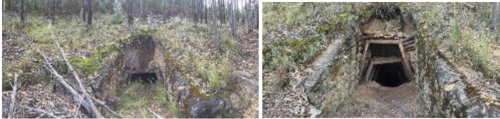
Before and after support stabilization
