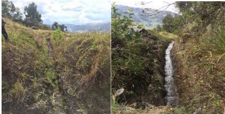
Before and after the coformation of the ditches for surface water management:
