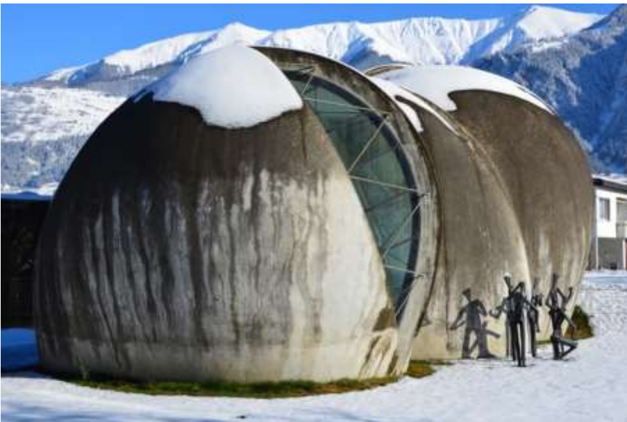
Figure 8 Shell construction of the stone church in Cazis (source: graubuenden.ch)
