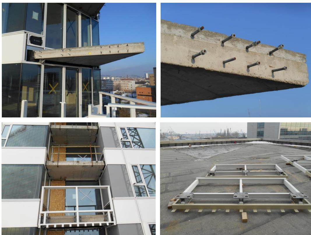
*Fig. 2 Anchor blocks and balcony railing with mounting brackets*
