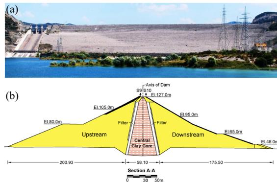
**Fig. 1** (a) Downstream shoulder of Pournari I dam with the concrete spillway (left) and part of the hydroelectric station (right). (b) Cross section of the Pournari I dam at the location where maximum height is obtained.
