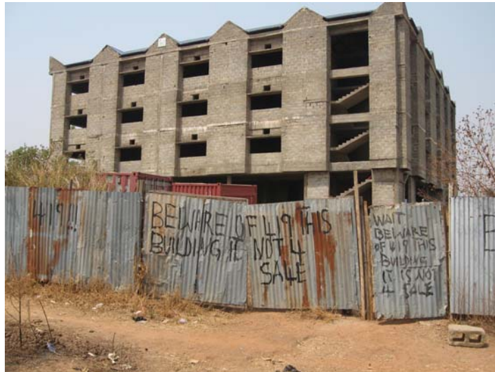
Figure 2 Notice on Wall to Deter Fraudulent “419” Transactions
