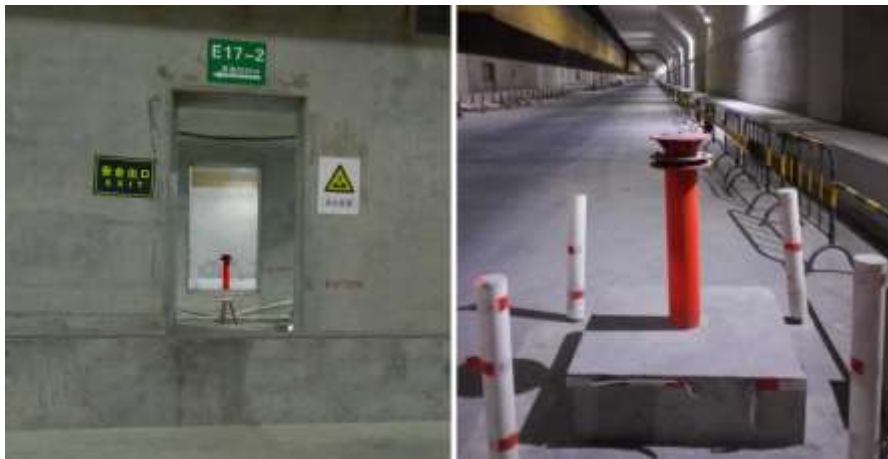
Fig. 6 Inter-visibility between the two bores and steel pillar with forced centering plate
